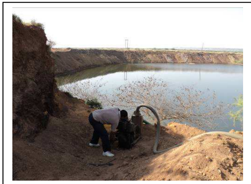
Setting up of pumping station
