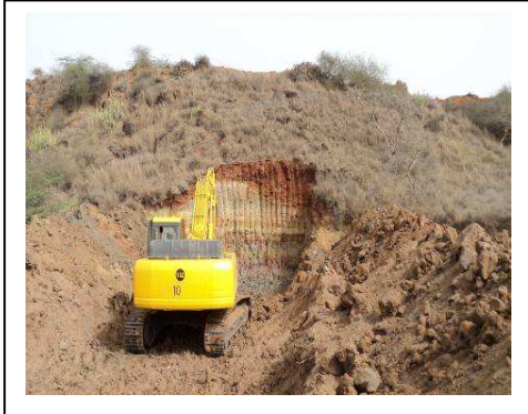
Site preparation for check dam
