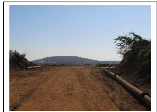
Gravity conduits heading towards inlet.
